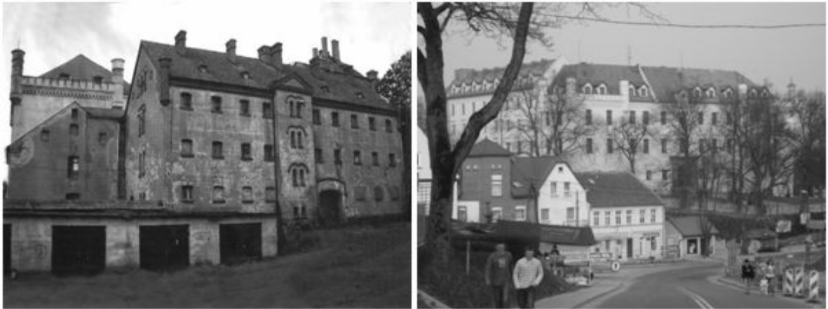
Figure 1 – View of the castle in Ryn before and after renovation.
